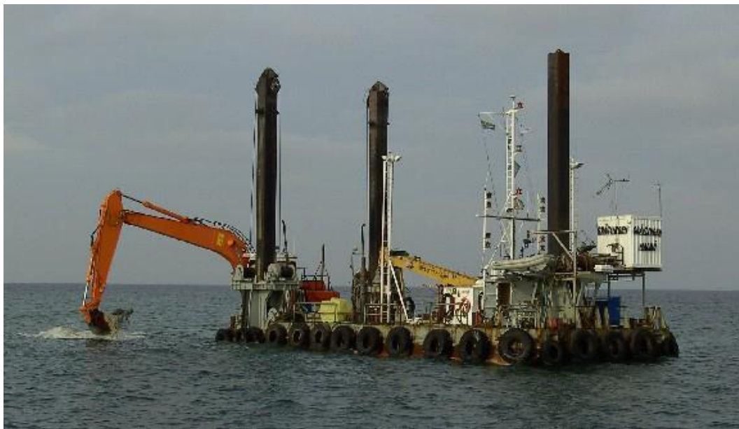
Fig. 1.2.3. Preparation of the seabed for laying a submarine cable (photo by Jeppsson et al. 2008).
