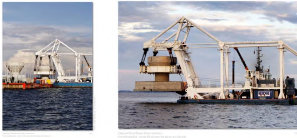
Fig. 1.2.2. Installation of WT foundation structures offshore (photos by Jeppsson et al. 2008).
